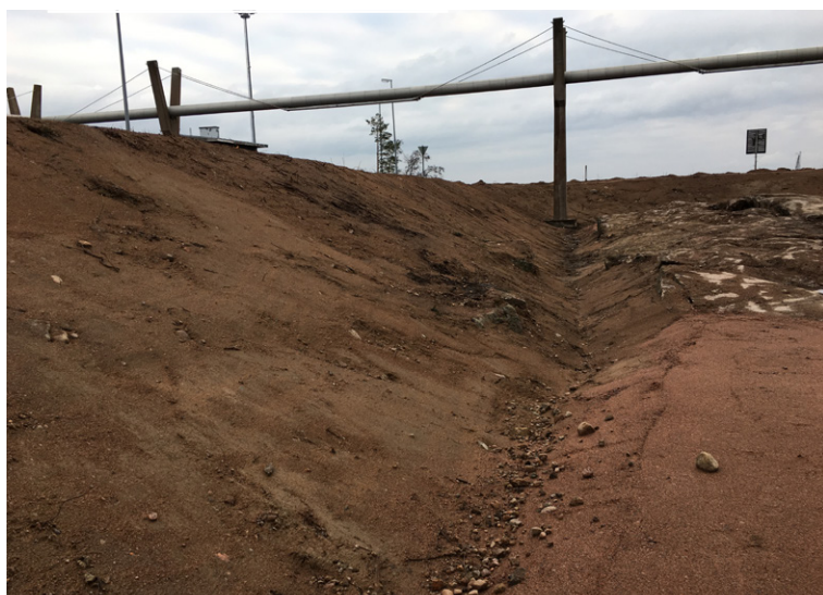
Bund following ground preparation works
