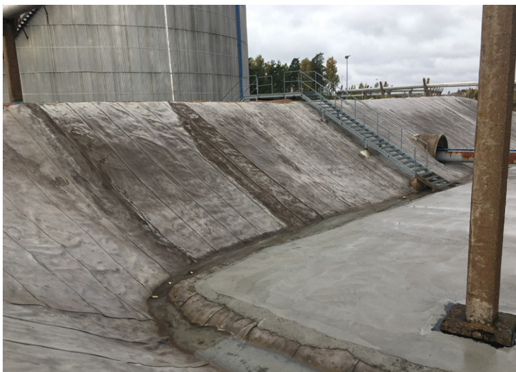
The completed bund installation
