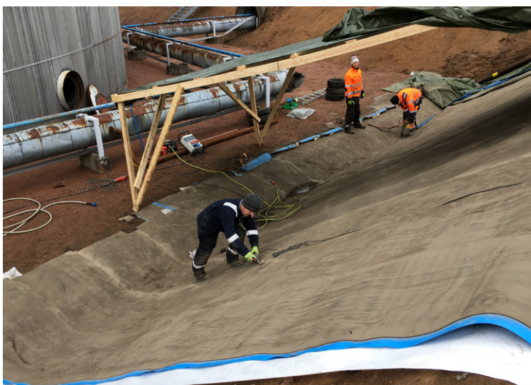
CCH thermally welded under makeshift canopy to keep material dry
