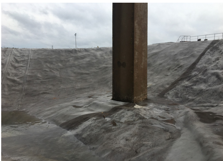
The CCH was cut to fit around existing infrastructure
