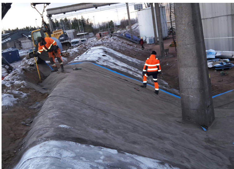
The CC was laid vertically down the bund slope
