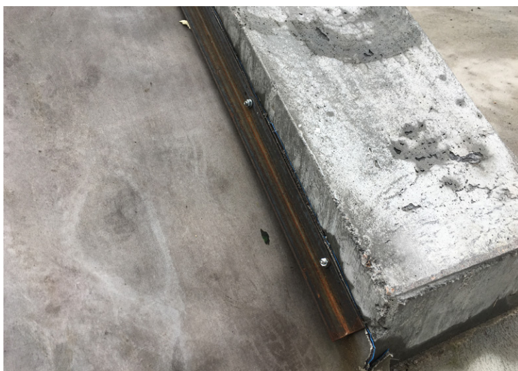
Steel bars and screws secured CCH edges against existing infrastructure
